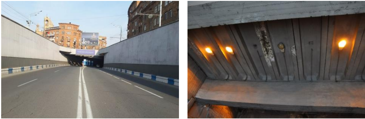
Picture 45: Enter to the tunnel from the Victory Bridge and its internal illumination system
