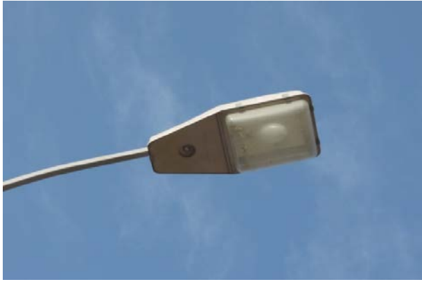
Picture 43: Typical old luminaries with 250W HPS lamps installed on the pilot streets in Ararat Region
