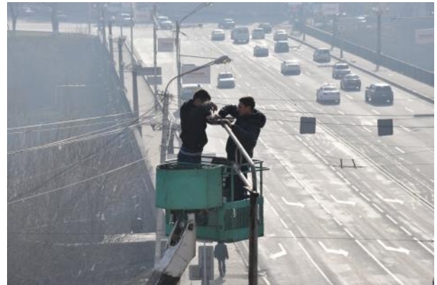
Picture 19: Installation and adjustment of new luminaries organized by YIC
