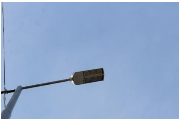
Picture 30: New 120W LED street luminary and night time view on the pilot street with the new lighting system
