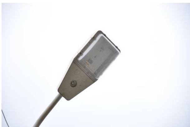
Picture 25: Old luminaries with 250W HPS lamps
