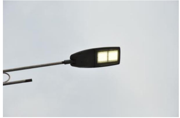
Picture 18: Old luminaries with 250W HPS lamps and new 213W LED luminary installed on Isakov Avenue
