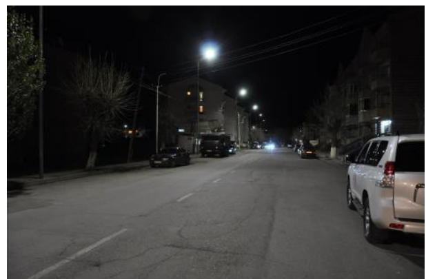
Picture 30: New 120W LED street luminary and night time view on the pilot street with the new lighting system
