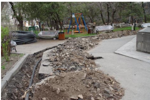
Picture 23: Installation of new feeding system and LED luminaries
