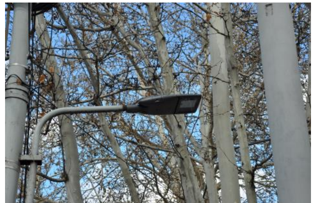
Picture 38: New 139W and 36W LED luminaries installed for street and sidewalk (Mashtots Avenue)
