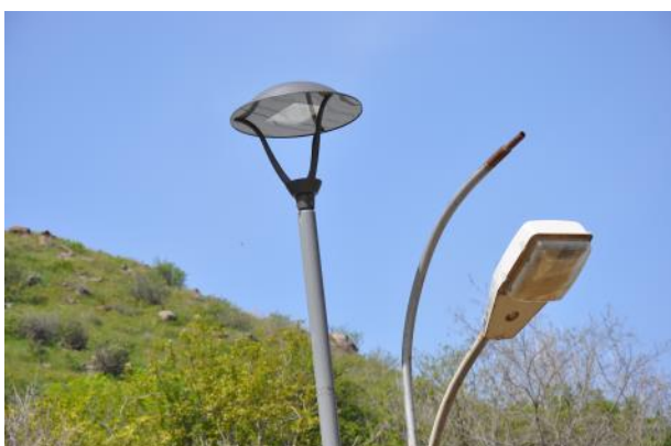
Picture 24: Installation of new feeding system and LED luminaries
