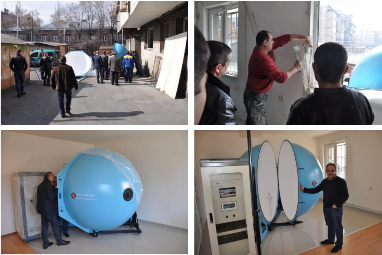
Picture 17: Installation of the equipment at the new laboratory premises provided by Yerevan Municipality
