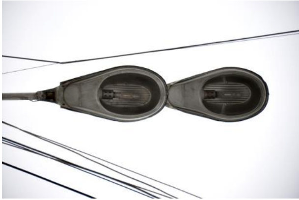
Picture 18: Old luminaries with 250W HPS lamps and new 213W LED luminary installed on Isakov Avenue
