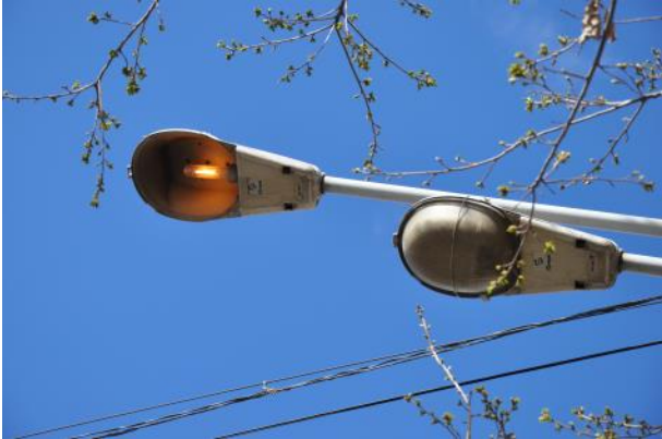
Picture 37: Old luminaries with 250W and 70W HPS lamps for street and sidewalk (Mashtots Avenue)
