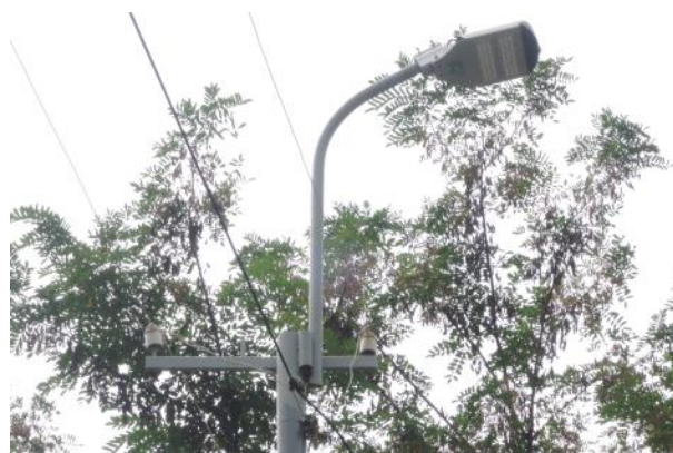
Picture 26: New 50W LED street luminaries installed under the pilot project
