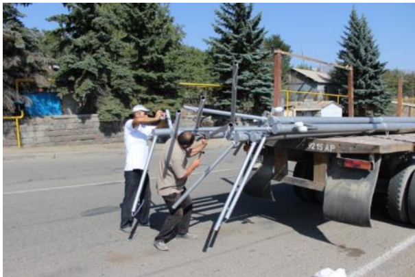
Picture 29: Delivery and installation of new lighting poles
