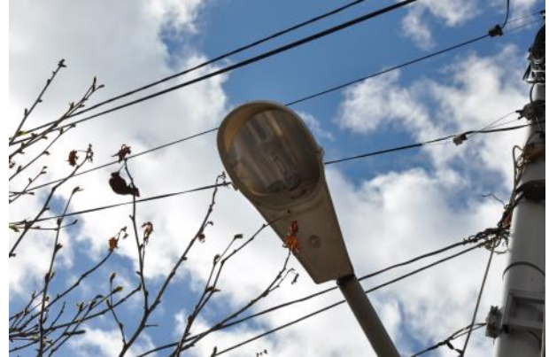
Picture 37: Old luminaries with 250W and 70W HPS lamps for street and sidewalk (Mashtots Avenue)
