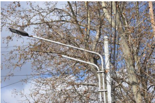
Picture 38: New 139W and 36W LED luminaries installed for street and sidewalk (Mashtots Avenue)
